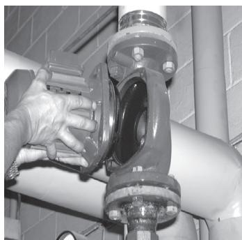
1) Detach the motor unit as usual (see Replacing motor and replacement motor unit).
