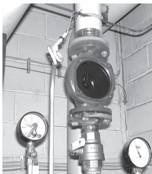
4) Replace the gasket/O-ring of the housing.
