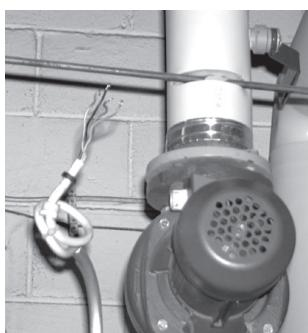
2) Detach the motor cable. Open the screws/bolts of the operating unit.
