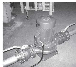
1) Stop the pump, open a possible safety switch and remove fuses. Ensure that no one is able to switch the current on, even by accident, during the replacement. Close the valves.
