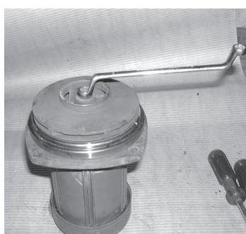
3) Open the screw/bolt of the impeller.
