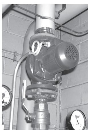
6) Connect the motor cable and open the valves. Start the pump and check the direction of rotation. Vent the system. Monitor the operation of the pump.
