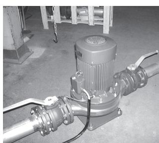
6) Connect the motor cable and open the valves. Start the pump and check the direction of rotation. Vent the system. Monitor the operation of the pump.
