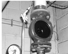
4) Replace the gasket/O-ring of the housing.
