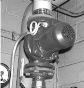
1) Stop the pump, open any possible safety switch and remove fuses. Ensure that no one is able to switch the current on, even by accident, during the replacement. Close the valves.
