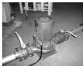
2) Close the valves and detach the connecting cable of the motor. Next, detach the flush pipe (in AKN\_H, AL\_H and L\_H - pumps). Open the screws/nuts of the operation unit.
