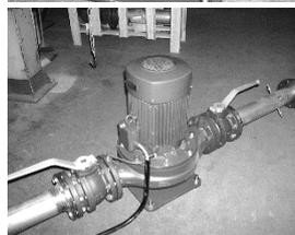
6) Connect the motor cable and open the valves. Start the pump and check the direction of rotation. Vent the system. Monitor the operation of the pump.
