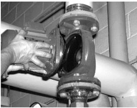
3) Lift the operation unit from the pump housing. Watch out for hot water!
