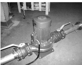
1) Stop the pump, open a possible safety switch and remove fuses. Ensure that no one is able to switch the current on, even by accident, during the replacement. Close the valves.
