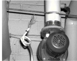
2) Detach the motor cable. Open the screws/nuts of the operating unit.
