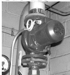
6) Connect the motor cable and open the valves. Start the pump and check the direction of rotation. Vent the system. Monitor the operation of the pump.
