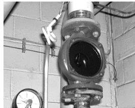
4) Replace the gasket/O-ring of the housing.
