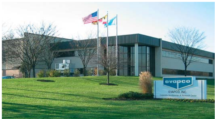
EVAPCO World Headquarters - Taneytown, Maryland, USA
