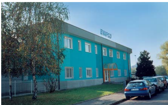
EVAPCO Europe Factory - Rho (Milano), Italy
