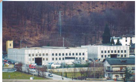
EVAPCO Europe Factory - Sondrio, Italy
