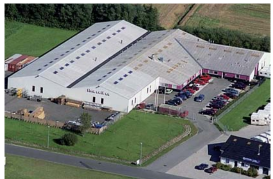
EVAPCO Europe Flex Coil Factory - Aalborg, Denmark
